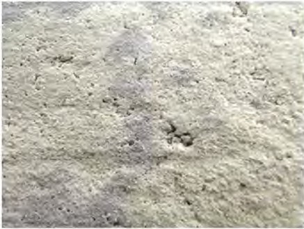
Cross section showing cavities.
